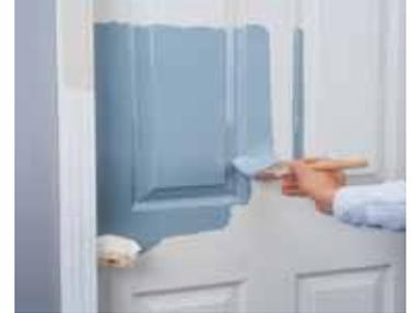
Spot prime all bare areas, including weathered, worn, patched or repaired areas, as directed above, followed by a spot coat of the finish coat paint to assure a more uniform appearance of the overall finish coat.
