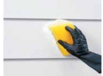
Bare or previously painted surfaces **must** be free of grease, wax, oil, soap film dust and dirt. Painting over grease, wax, oil and soap film will cause poor drying and curing of the paint film, and poor adhesion. Dull glossy finishes by sanding lightly.
