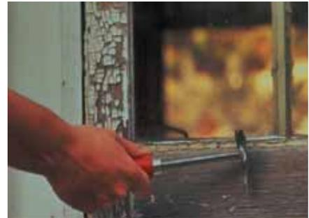
Preparation for painting interior walls, ceilings and woodwork is relatively easy and the few paint failures which occur on these surfaces are generally attributable to failure to remove grease and wax and to dull glossy surfaces. If the following preparation instructions are followed, the incidence of interior wall paint failure is dramatically reduced.
